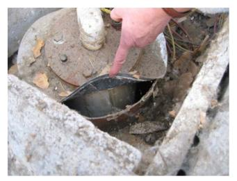
Seal on wellhead not watertight
