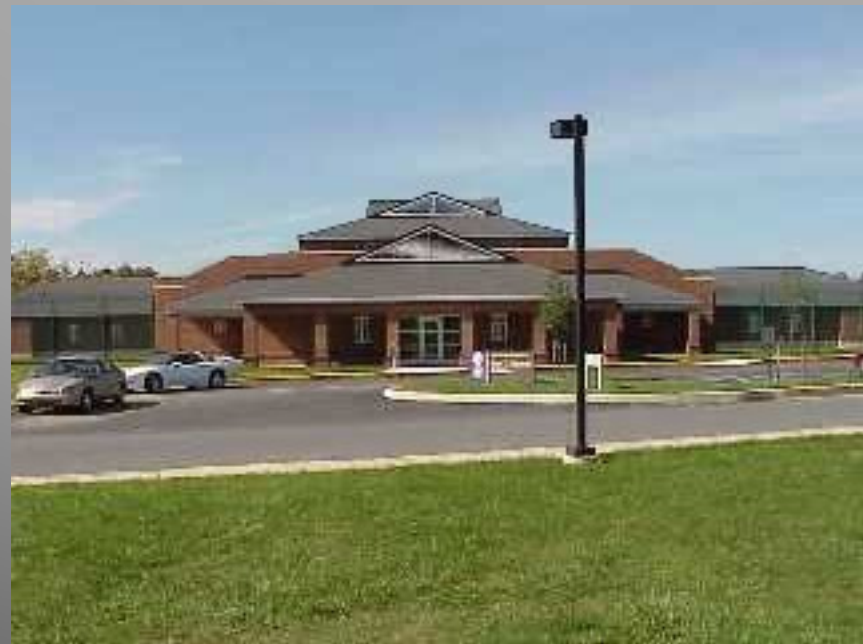
Mitchell Building, Holloway Campus
